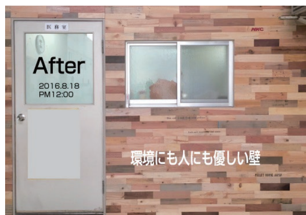
Examples of waste pallets reused as external wall decorations
