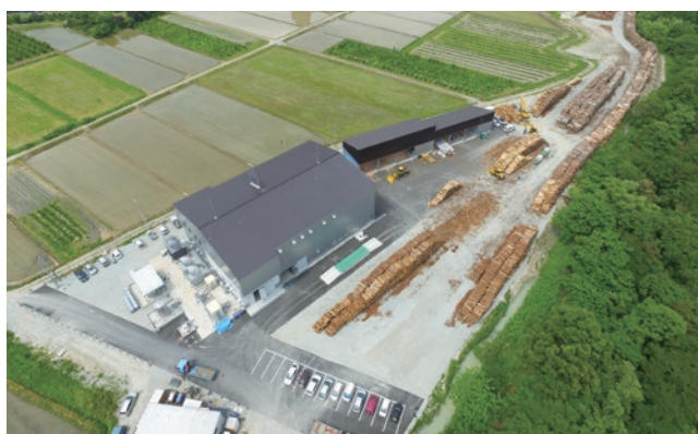
Nagai Power Plant
