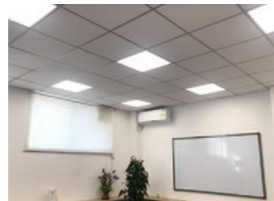
Shifting to LED lighting fixtures
