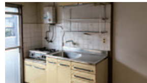
Remodeling (before renovation)
