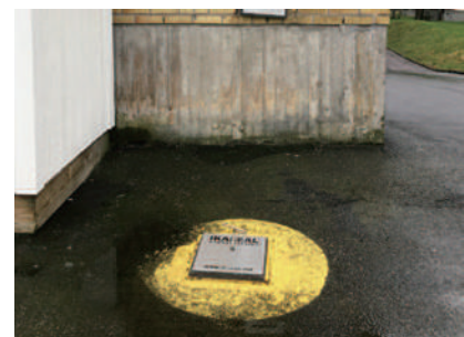
Cover for prevention of effluent leakage
